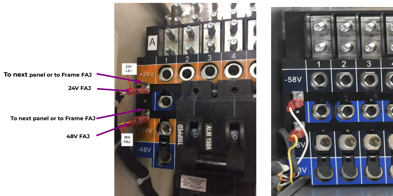
Figure 24 Breaker Panel Alarm Connections
